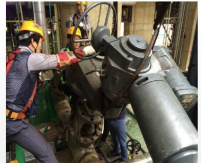
The VALVE MEDIC TEAM (valve maintenance organization) is repairing the MOTER OPERATED VALVE.
